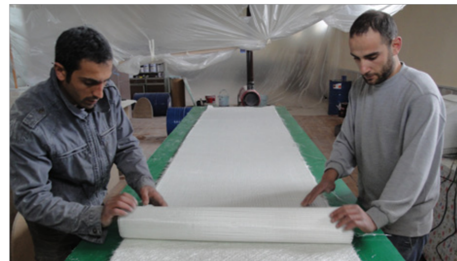
Layup of METYX Composites fabrics into the L-RTM mold
